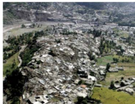
Above: Aerial view of devastation caused by EQ 2005- Balakot City, KPK
